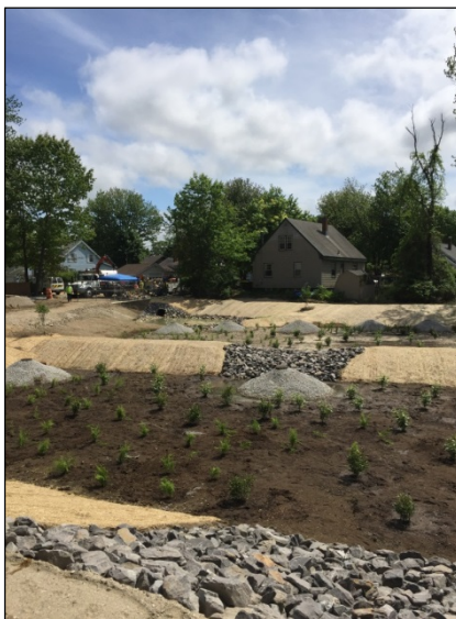
Gravel wetland installed in South Portland in 2016 with CWSRF
