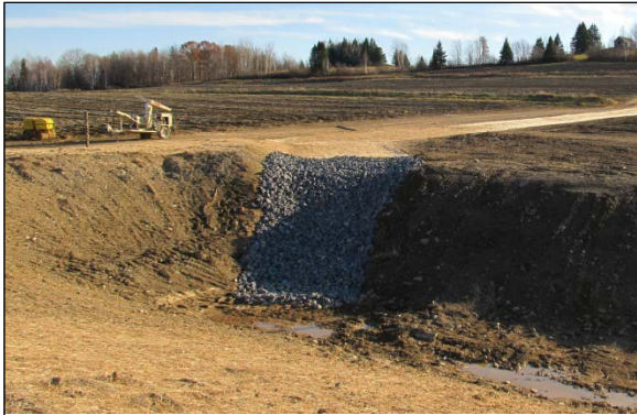
Sediment basin with grass waterway
