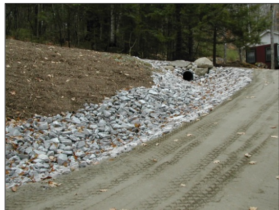
Merganser Lane – After BMP Installation
