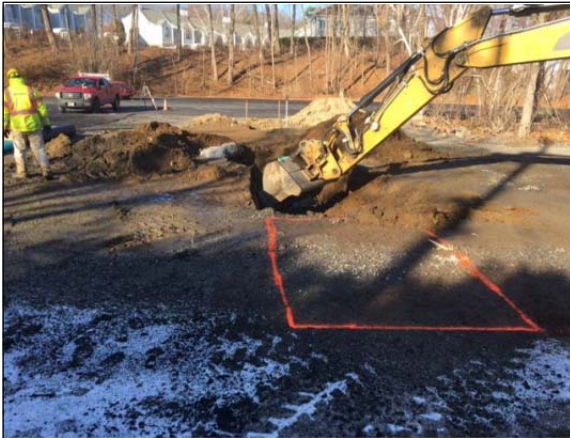
Installation of bio-retention unit to treat the runoff from the Ogunquit Lower Parking Lot
