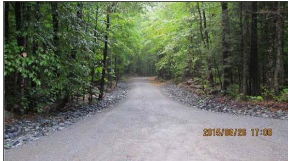
Granite Estates - bluestone gravel and ditching turnouts
